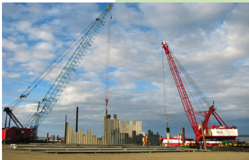
Port of Anchorage Intermodal Expansion Project DOT, Maritime Administration Contract
