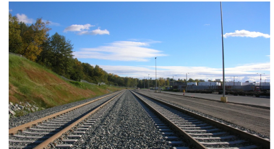
Railway Extension - Construction Management & Professional Engineering Services Provided by ICRC
