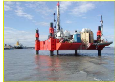
The Jack-Up Rig at high tide
