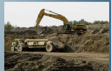
Excavation at the North End Borrow Pit
